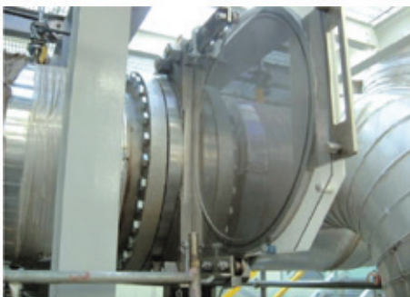
Heat exchanger - Bypass line
